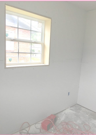
Sheet Rock Installation in Progress
